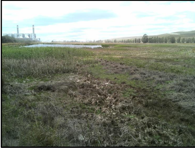
Figure 13. Earthworks and existing dams.
