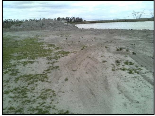
Figure 14. Earthworks and existing dams.
