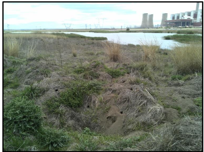
Figure 16. Earthworks and existing dams.
