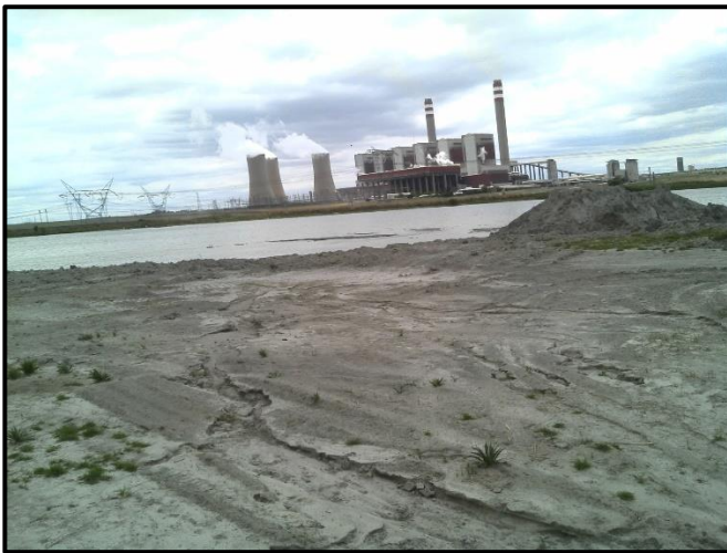
Figure 15. Earthworks and existing dams.
